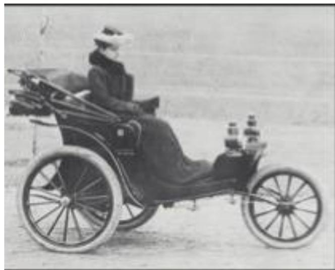
*Rhea Duryea Johnson, oldest daughter of Charles E. Duryea, at the stick of an early three-cylinder Reading Duryea. The stick in the left hand steered the car, shifted gears and accelerated this snappy model. Three operations in one followed Duryea's idea of simplification for the driver*
